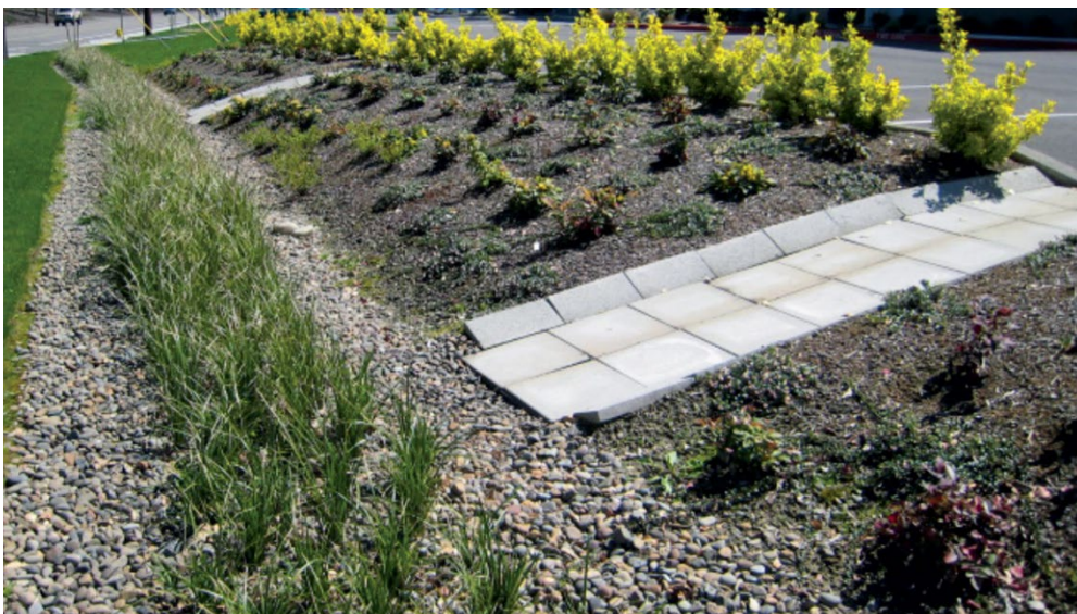
RAIN GARDEN AT SACRAMENTO STATE
